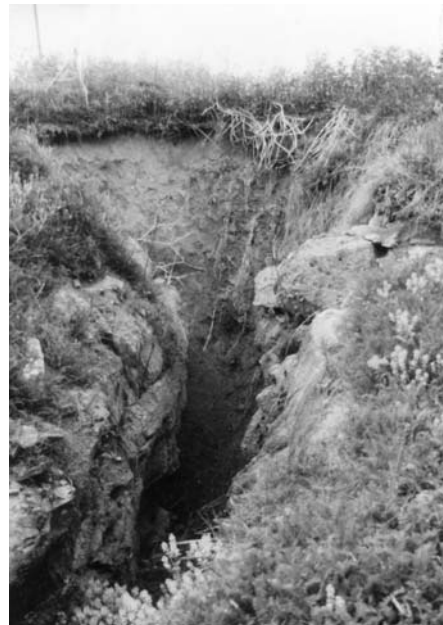
Figure 11. A sinkhole having an open drain.
