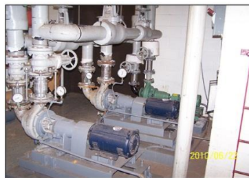
Photo 6 - Existing Heating Hot Water Circulating Pumps
